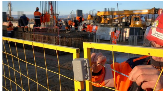
Fig. 1. An example of a dangerous employee moving.
